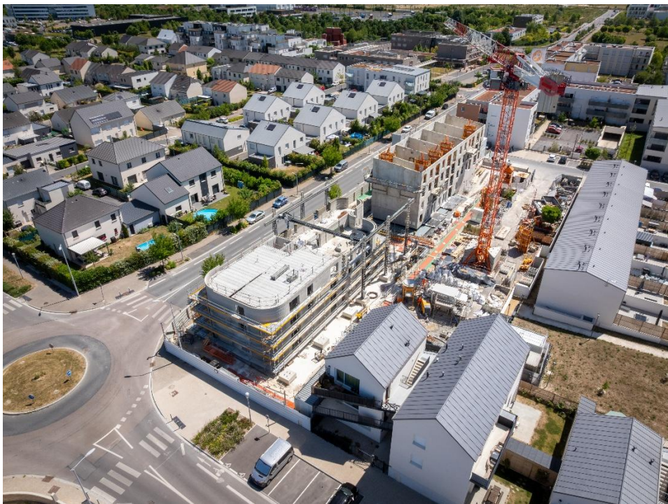
ViliaSprint 2 - ©PERI 3D Construction
